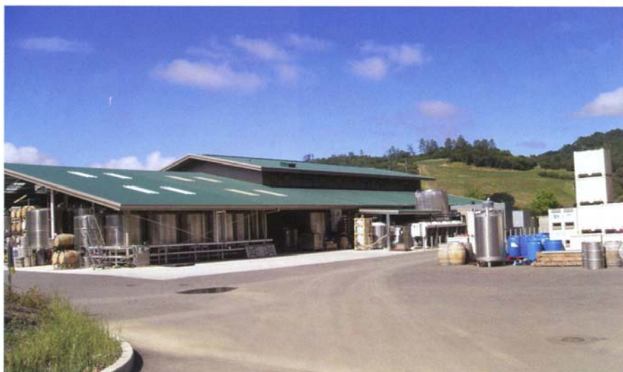
Somerston's owners opted to invest in technology to improve the winery's energy efficiency, instead of spending money on aesthetics or LEED certification.
