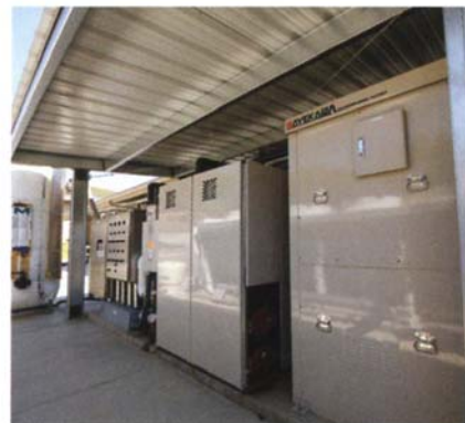
The Mayekawa Eco Cute heat pump uses CO 2 to simultaneously cool glycol and heat hot water. Photo: Craig Lee
